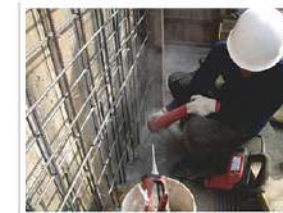
Concrete wall addition
