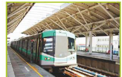
■ Kaohsiung Rapid Transit Construction Project.
