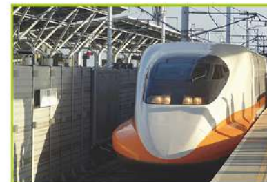
■ Taiwan High Speed Rail Miaoli Station Construction Project.
