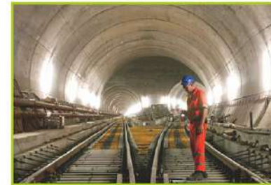
■ Tunnel Construction Project.
